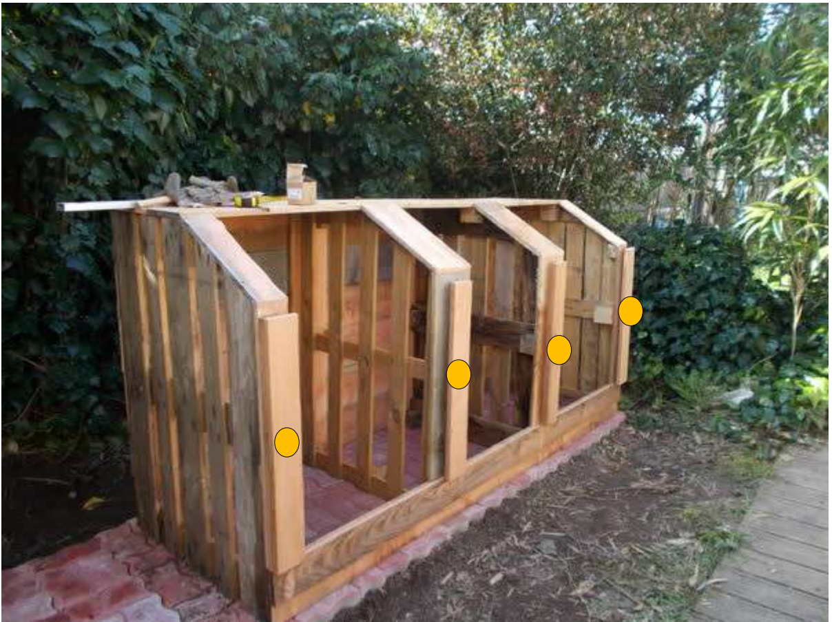
Runners between each containers so as to easily put in or take out planks and simplify its use. At the bottom of the runners, there is a stop that holds the planks.
