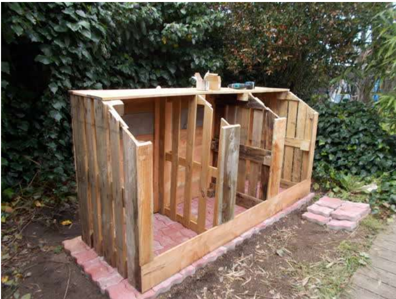
Compost container made with pallet wood and second-hand Douglas wood.
