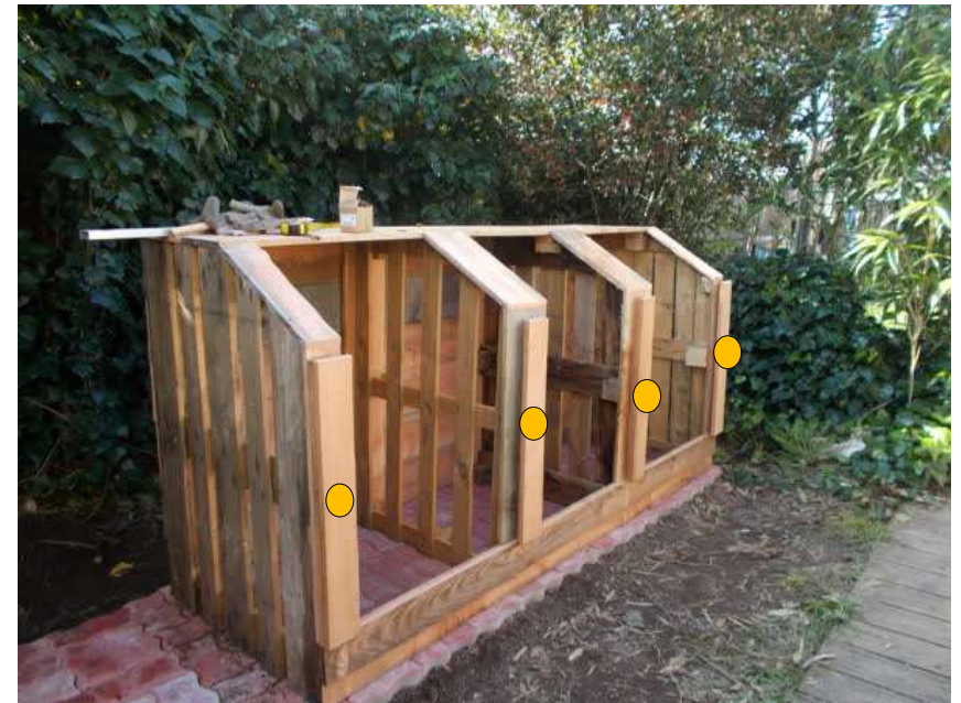
Runners between each containers so as to easily put in or take out planks and simplify its use. At the bottom of the runners, there is a stop that holds the planks.
